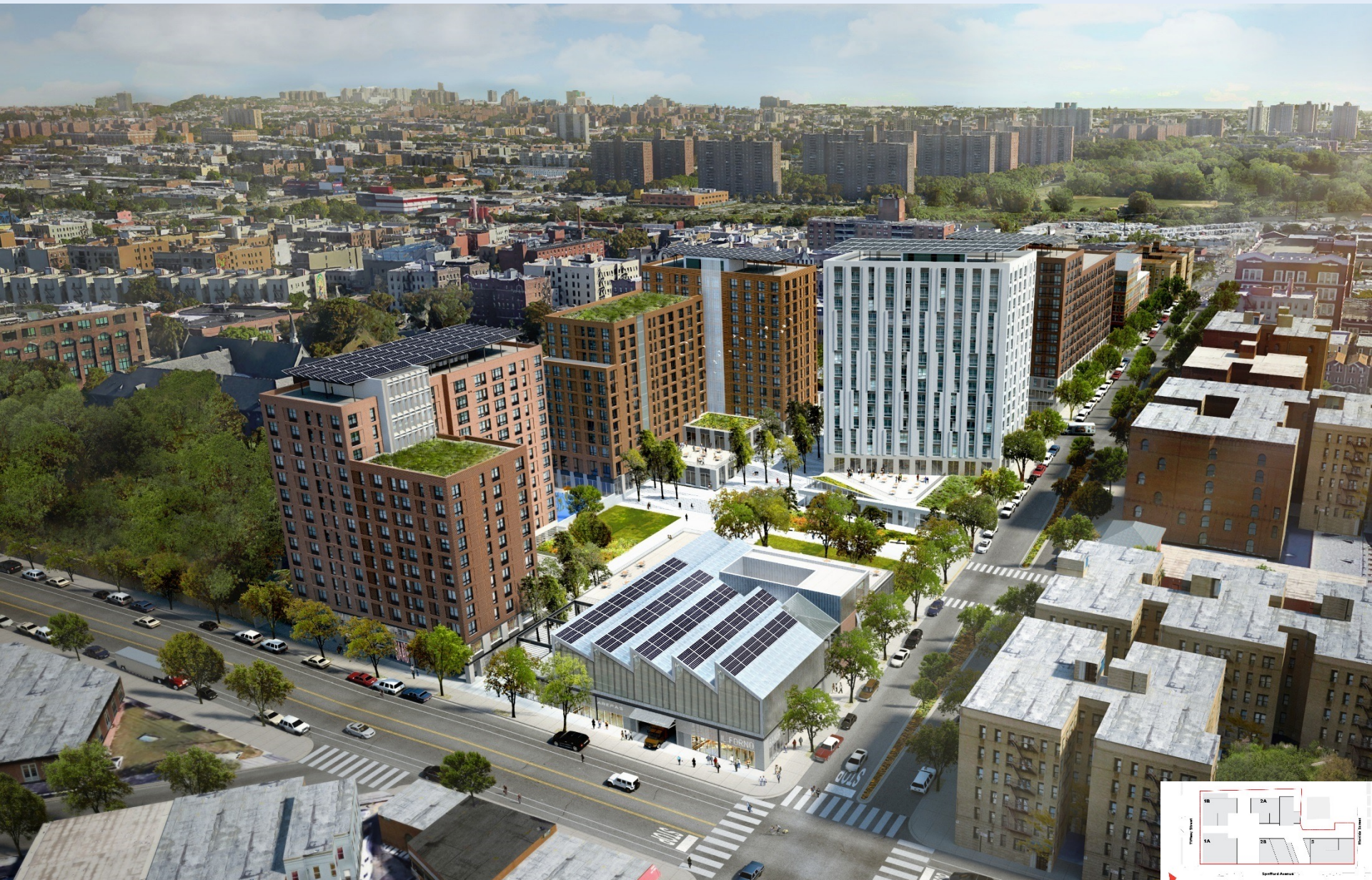
AERIAL VIEW FROM SOUTH WEST
